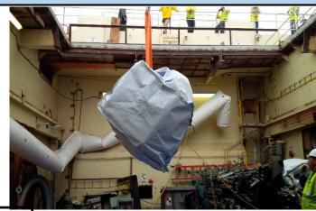
The hatch cover was lifted and the items were removed from the upper refueling room floor. The spent fuel rod transfer cask and the spent control rod transfer cask were packaged in supersacks (white bags) and then loaded into intermodals for truck transportation to the disposal facility.
